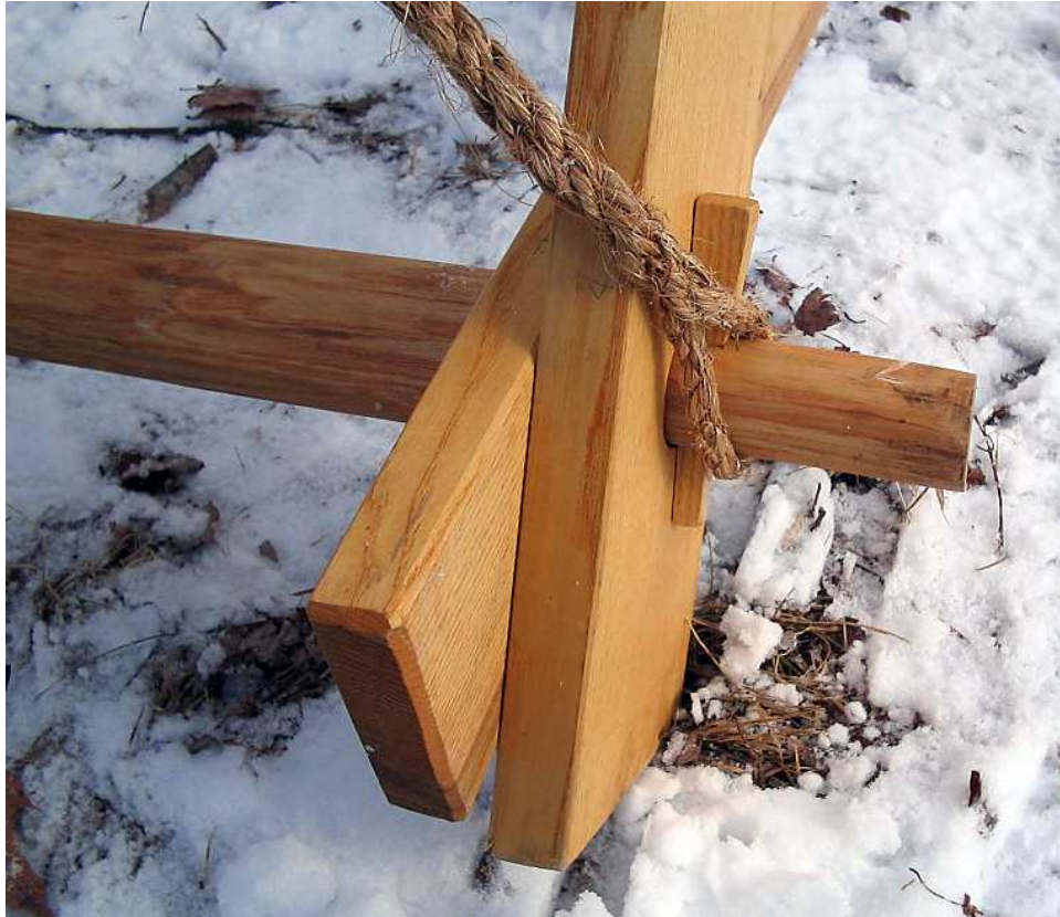
Detail showing ground pole passing through the shear leg and transom, with rope brace and peg
