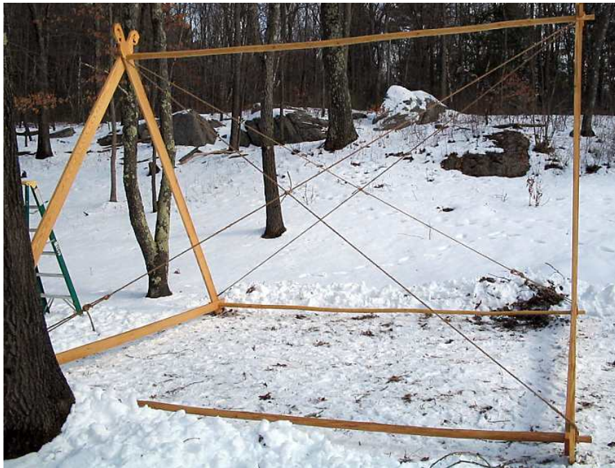
Tent frame showing the rope braces
